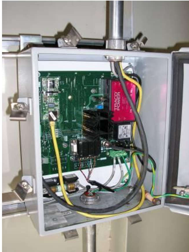
Figure 7 EFREM Receiver Mounted on Exciter Cubicle Wall
